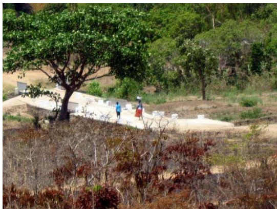
The bridge in use
